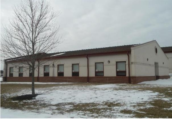
Runoff from the southernmost roofs of the building could be routed to bioretention systems. Downspouts could be fitted to downspout planter boxes. Multiple parking spaces could be repaved with pervious pavement. A preliminary soil assessment for this site suggests that the site's existing soils have suitable drainage characteristics for green infrastructure.
